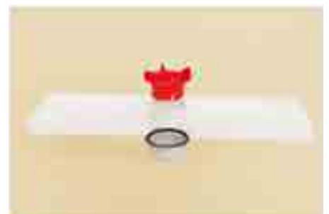
12. Insert the waste valve and screw it together with the counternut. The gasket has to be tight on the bottom of the tray
